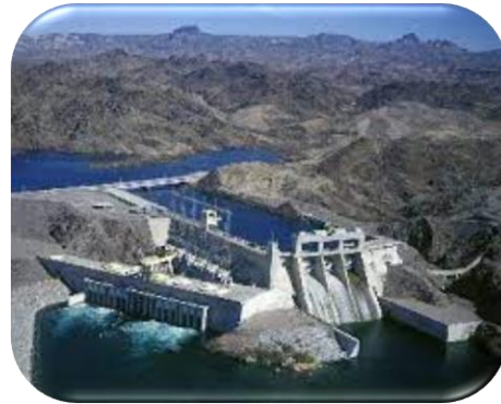
Bureau of Reclamation's Davis Dam (right) and the DeCew II Generating Station operated by Ontario Power Generation (left).
